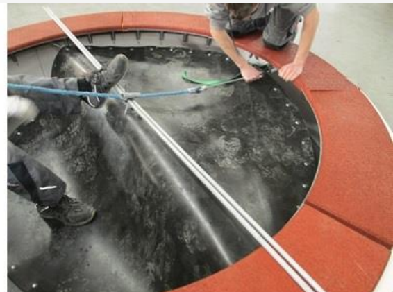
Fit tensioning strap 90 ° offset and opposite spring Hook.
